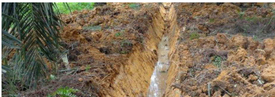
Figure 13. 'V' Shaped drain at BOPP.
